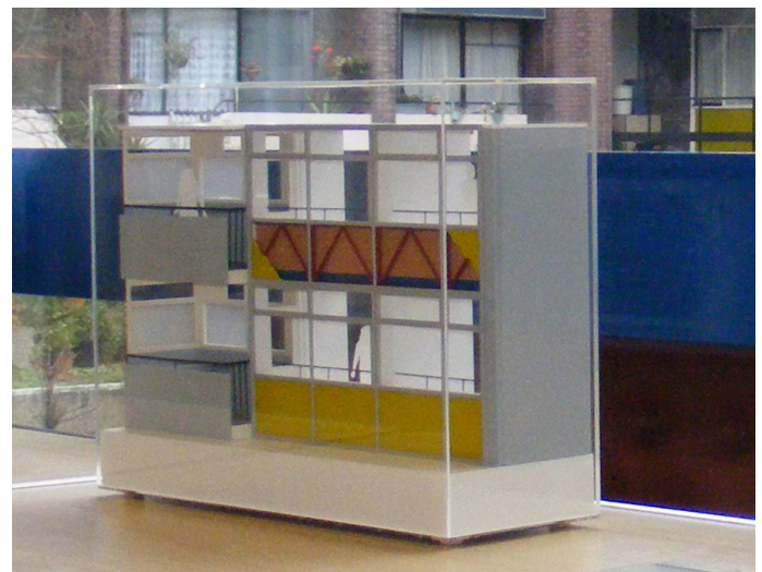
A 1:20 scale model of a typical proposed cladding module
